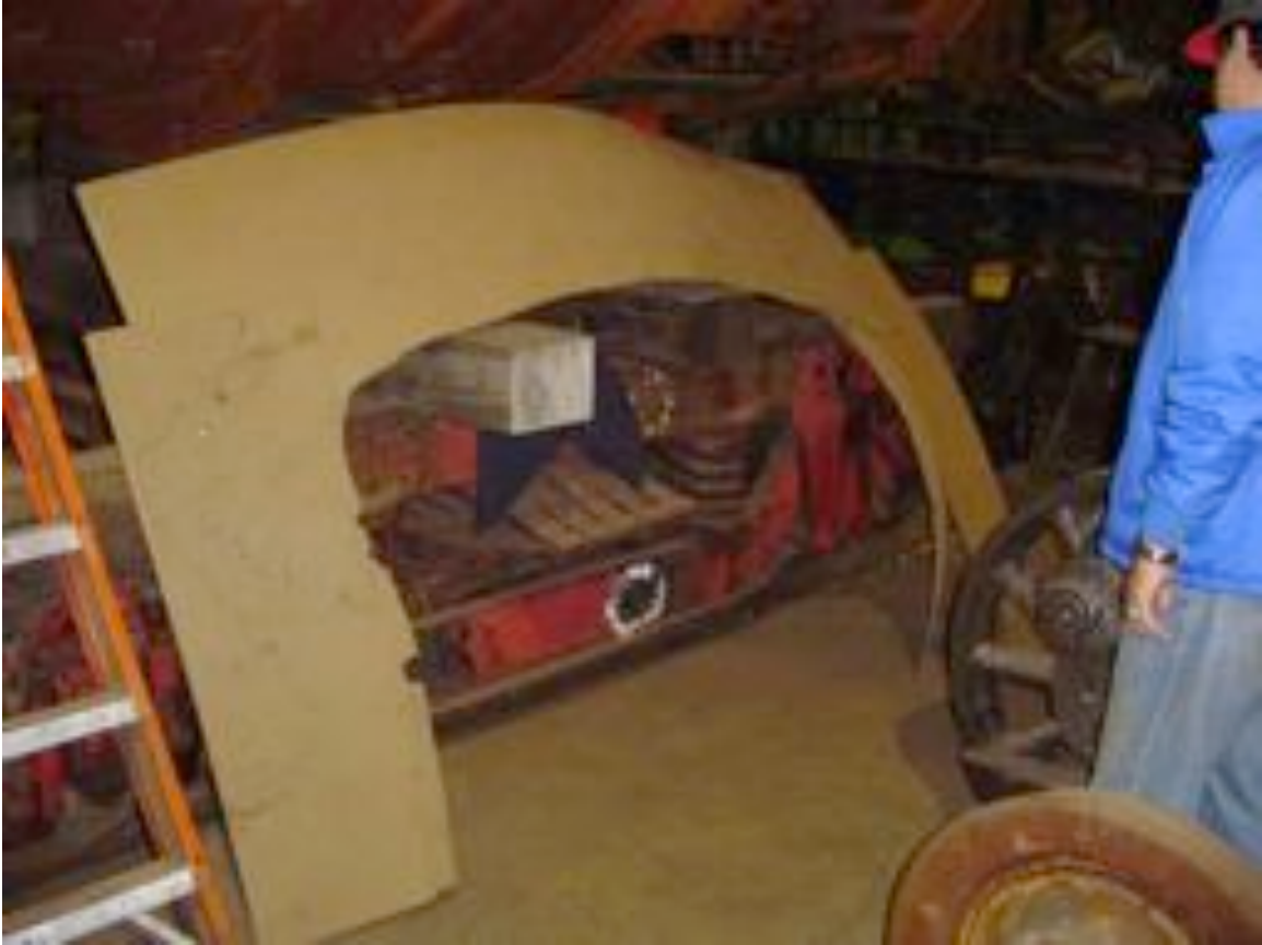
Before the roof and side sheets were removed, Masonite templates were made to assist in the formation of the new side sheet material and roof sheet.
